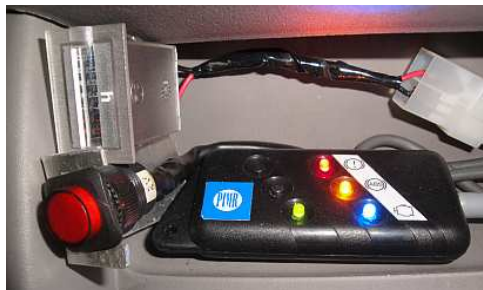
Fig. 29. L200 - LEDs control panel, counter of work hours of air compressors, red push button – trailer’s emergency braking action
