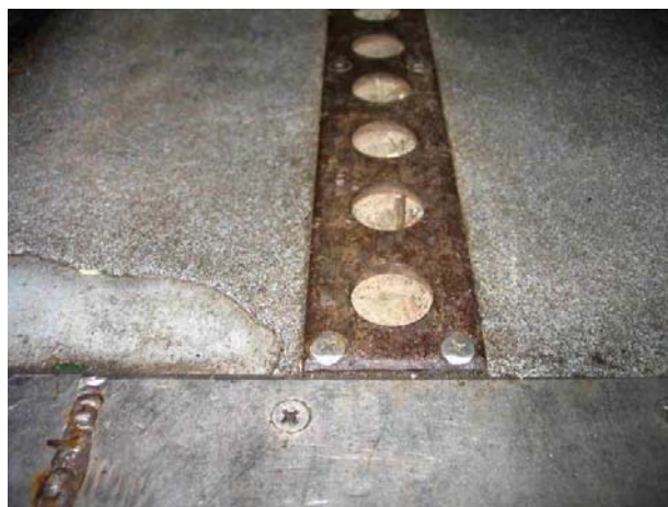
Fig. 8. Strengthening for the load protecting system sunk in the floor
